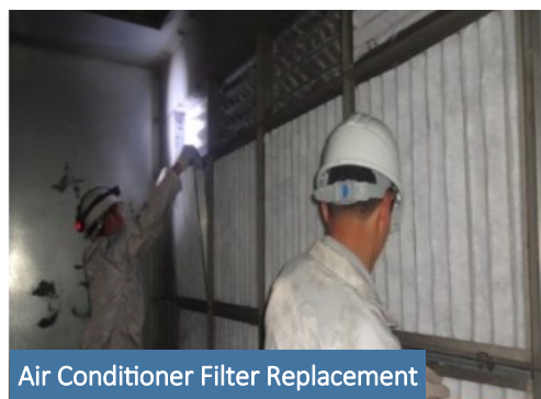
Clean the Air Conditioner Filter
